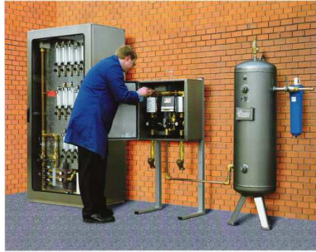
Milk powder processing, high flow gas mixer and distribution system
