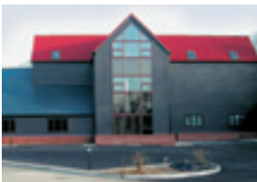
Sauer UK, Colchester Sales and Service office in United Kingdom
